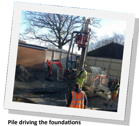
Pile driving the foundations
